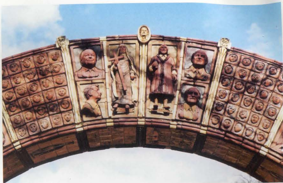
above: Detail of the uppermost tile on the Millennium Arch.
